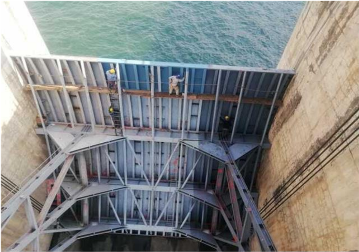
The spillway gate of Pong Dam
